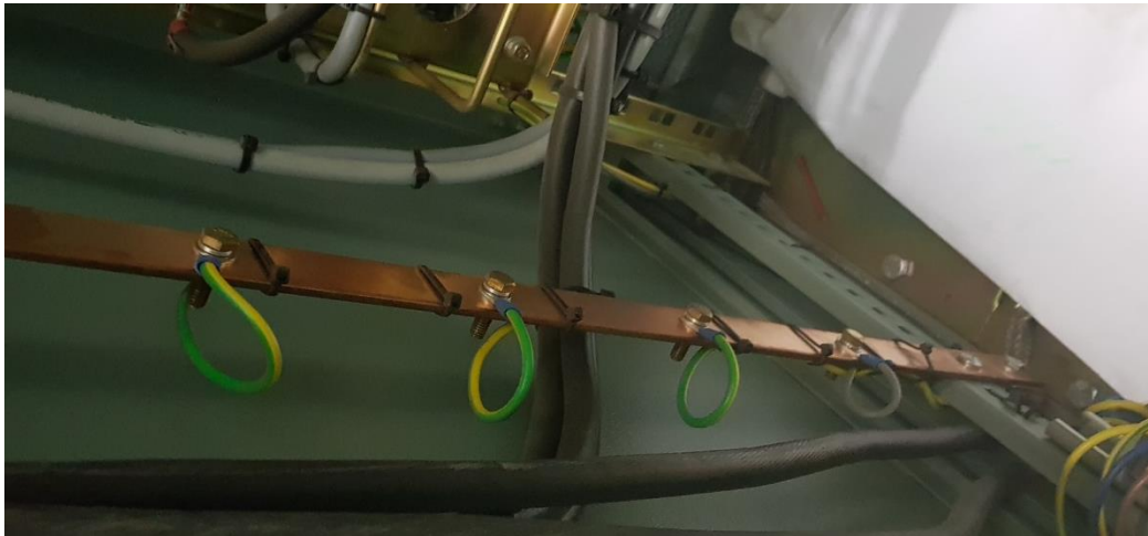
Figure 4: Cabinet earthing bar
